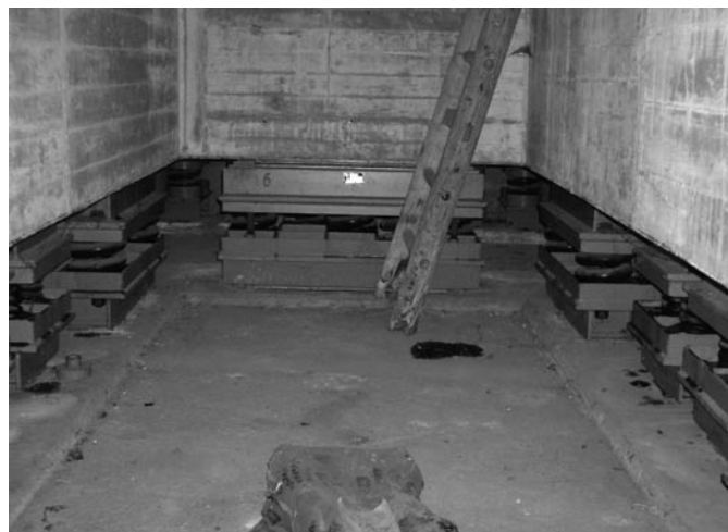
The complete house rests on springs designed by GERB
