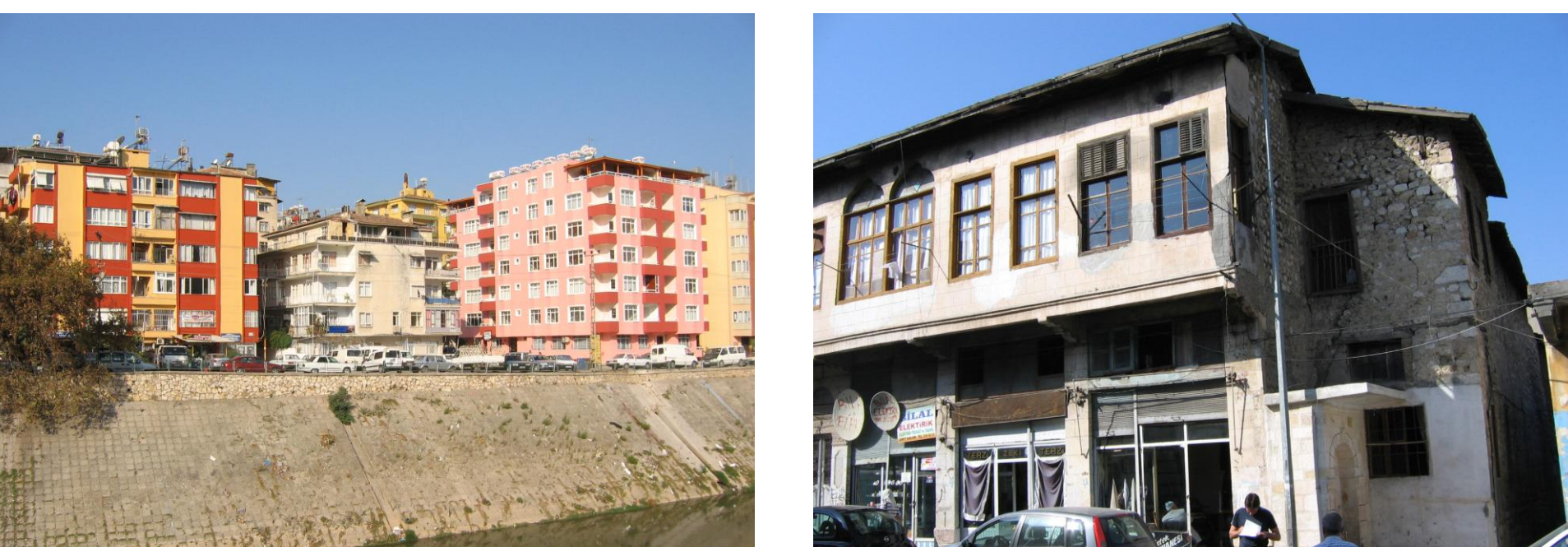
Figure 3.3. Examples of typical building types in Antakya: RC frame structures (left) and simple stone masonry structures (right)
