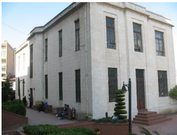
a) View of the instrumented municipality building
