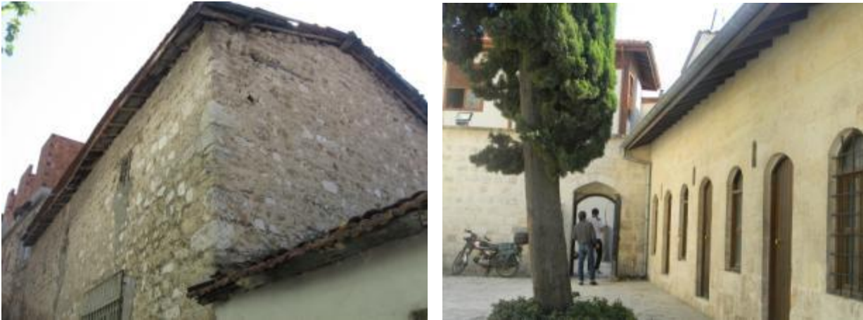
Figure 4. Surveyed stone masonry buildings; a) simple stone, b) massive stone
