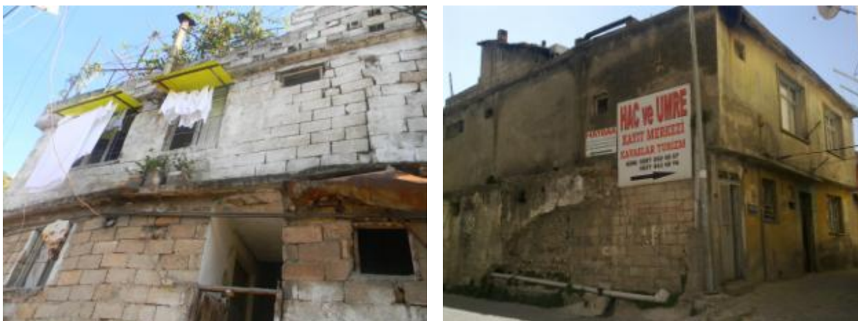
Figure 3. Surveyed masonry buildings constructed with cellular concrete blocks
