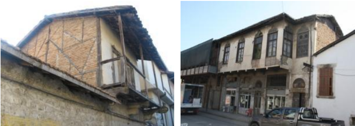
Figure 5. Traditional timber-laced masonry buildings called as “hımış”
