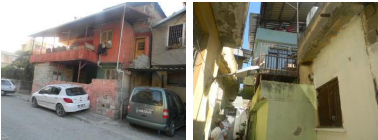
Figure 7. Surveyed masonry buildings with irregularities in elevation
