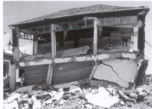
B2 Stahlbeton-Skelettbau in Düzce
