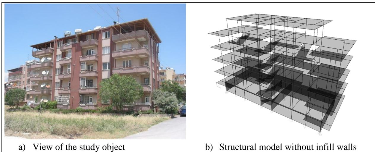
Figure 5. View and structural model of the example 5-story residential reinforced concrete building.
